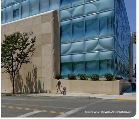
The two-layer glass façade, featuring *Starphire®* glass by Vitro Architectural Glass (formerly PPG glass), provides aesthetic and performance advantages to the recent renovation of the Gores Group World Headquarters, and plays a critical role in modulating the building's indoor temperature and air quality.
