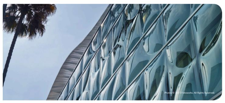
Starphire® glass by Vitro Glass in combination with carved limestone helped transform a non-descript three-story building into the stunning Gores Group World Headquarters. The façade is composed of three double-paneled, bent-glass patterns with a dozen different custom-printed interlayers sandwiched in between.
